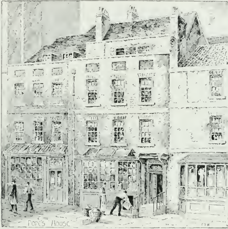
"POPE'S HOUSE" IN PLOUGH COURT, LOMBARD STREET, IN 1800.
